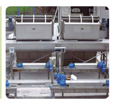
The sub-vertical mechanical bar screen SAVI GVB is used for coarse screening in municipal and industrial wastewater plants.
